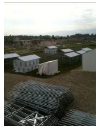
HODR's modular structures
